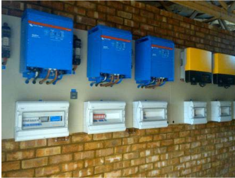
Blue inverters to power the 3-phase solar powered school
